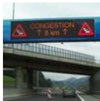
Variable message signs VMS LED
