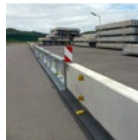
Temporary crash barriers
