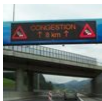
Variable message signs VMS LED
