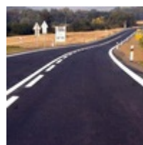
Horizontal road markings
