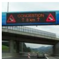
Variable message signs VMS LED
