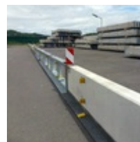
Temporary crash barriers
