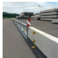
Temporary crash barriers
