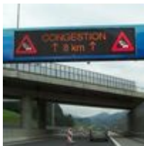
Variable message signs VMS LED
